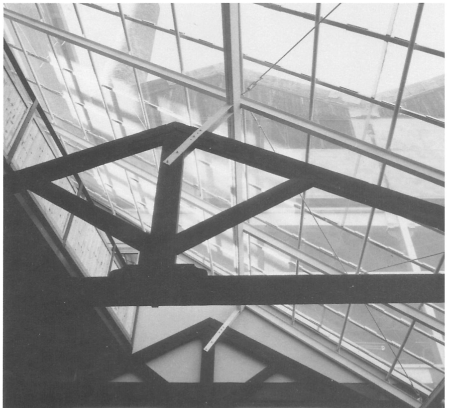
25. View through the glass roof
