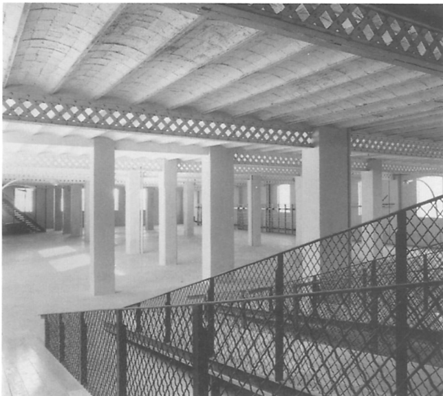
10. View of the ramps
