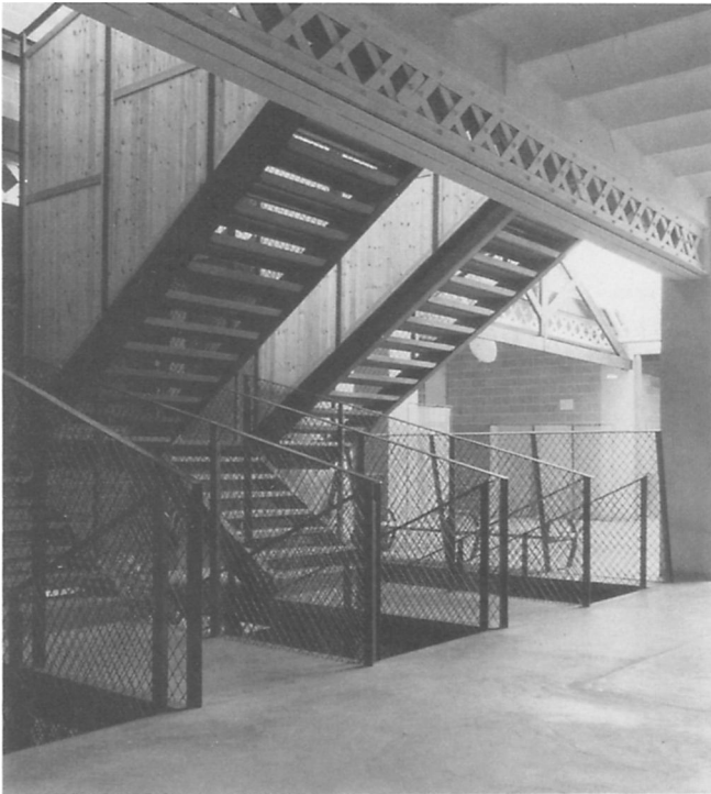
13. View of the stair
