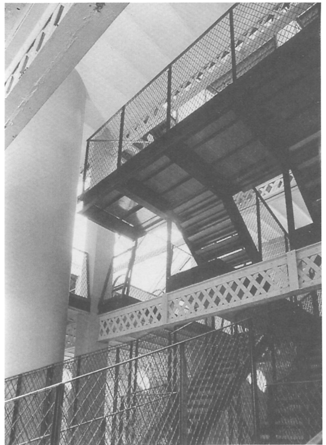
14. View of the stair
